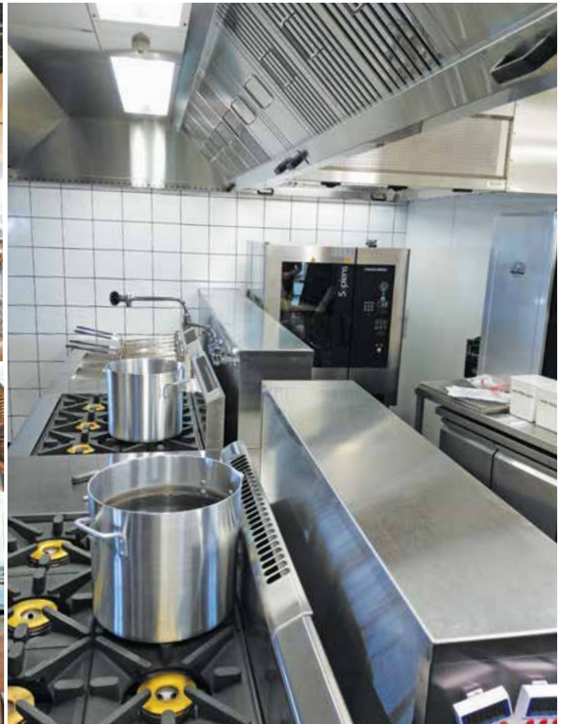
PROJECT SUPPLIED BY SOUTHERN HOSPITALITY, HAMILTON
